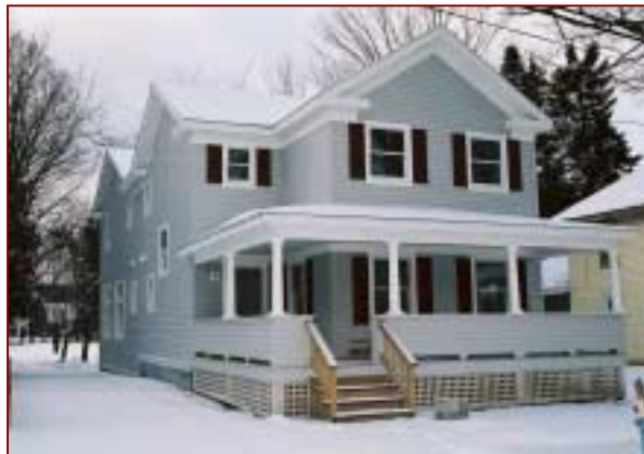
Photo: Exterior reconstruction complete. February 2002.
